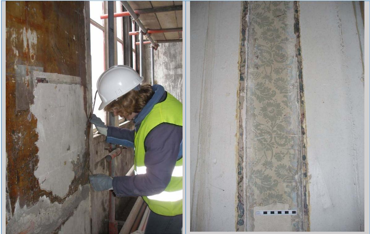
**Figure 1:** The Author retrieving wallpaper from St Pancras Chambers (Left), and the William Morris Venetian pattern wallpaper (right) as found in situ when a partition wall was removed. Another fragment of paper can be seen either side of it.
